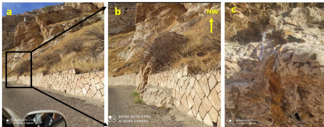
Fig. 11: Station (6), (a) Side view of the station. (b) Part of the station showing part of the retaining wall destroyed by blocks falling from the upper part. (c) The chert veins showing a thickness of 7.0 cm.
