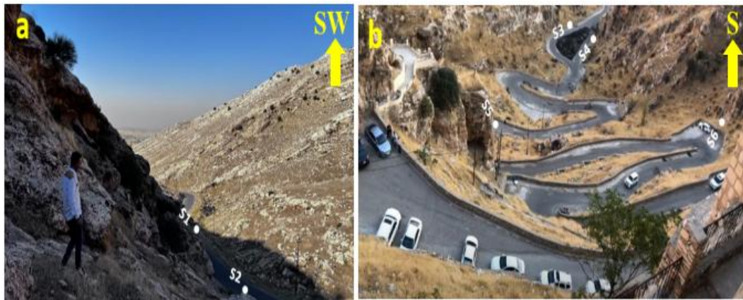
Fig. 3: Location of stations (a) the stations before the Monastery Gate taken from the top of the second station, (b) the stations after the gate taken from the top of the monastery terraces.
