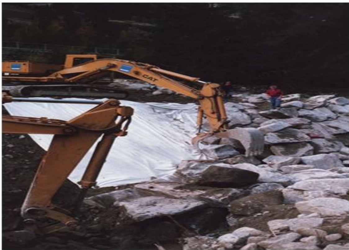
Fig. 12. Riprap with blocks of 4 to 4.5 t individually laid by a machine atop a geotextile functioning as a filter (Jafarnejad et al., 2019).
