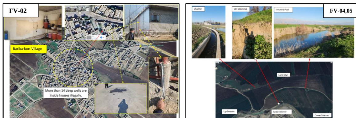
Fig. 17: Infrastructure deformation in Barika Kon town due to excessive well drilling, and subsidence effects in Kazhaw village (irrigation channels), Arbat, Halabjai Taza, and Nasser Camp (schools, mosques, and residential buildings).
