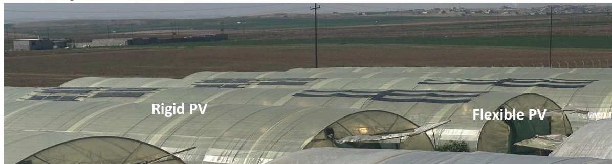
Figure (1): Installation of flexible and rigid PV panels on greenhouses roofs
